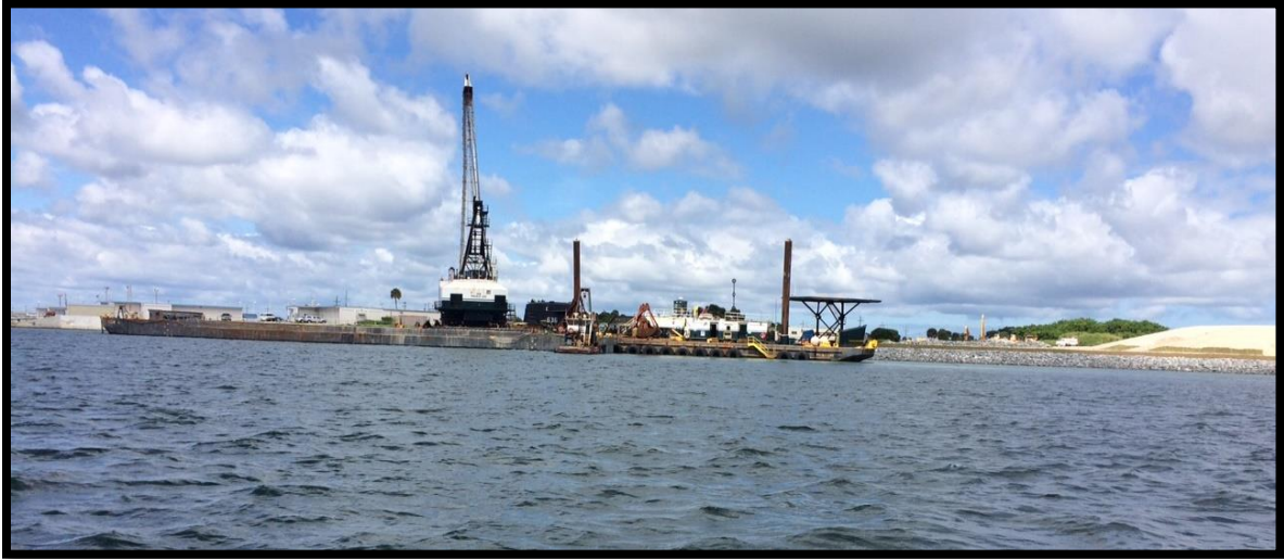
Figure 3. Example of construction activities in the area.
